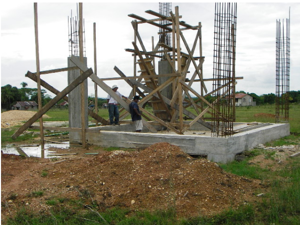
Water Suply Tank being built
